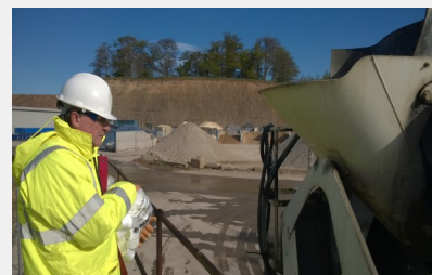
Adaugarea fibrelor in autobetoniera
